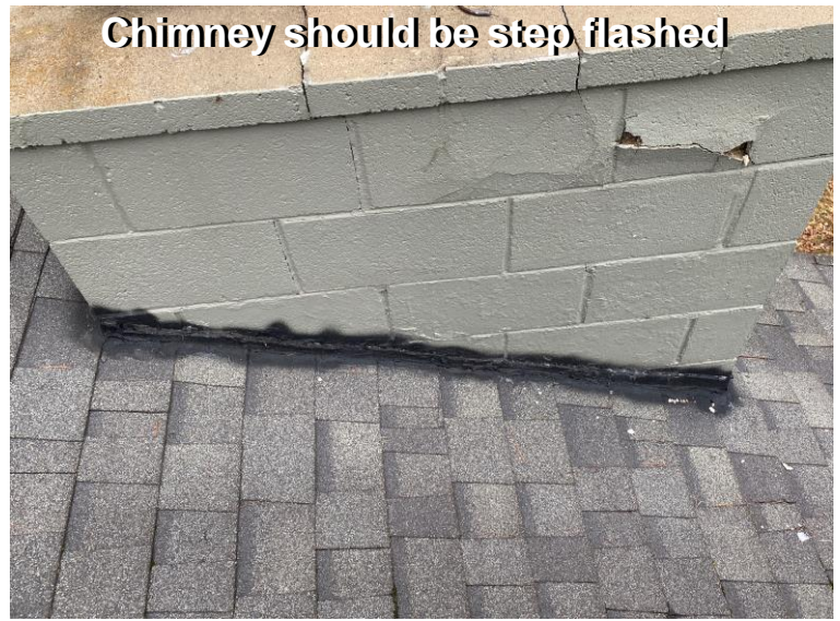
Chimney block deteriorating.
