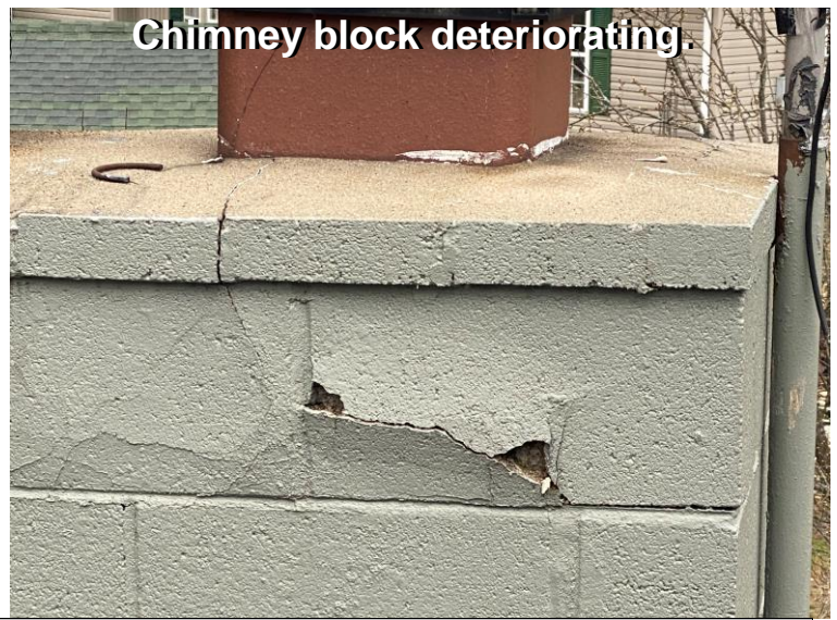
Flue liner deteriorated. Chimney cap cracked.
