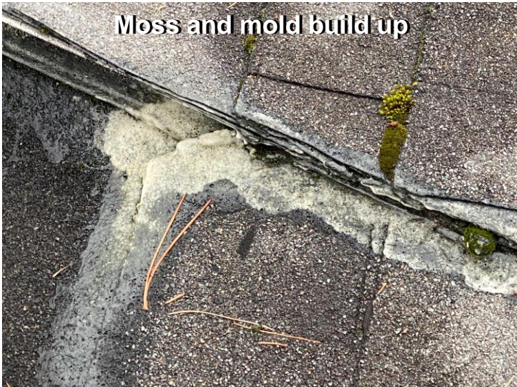
Valley holding moisture causing mold growth
